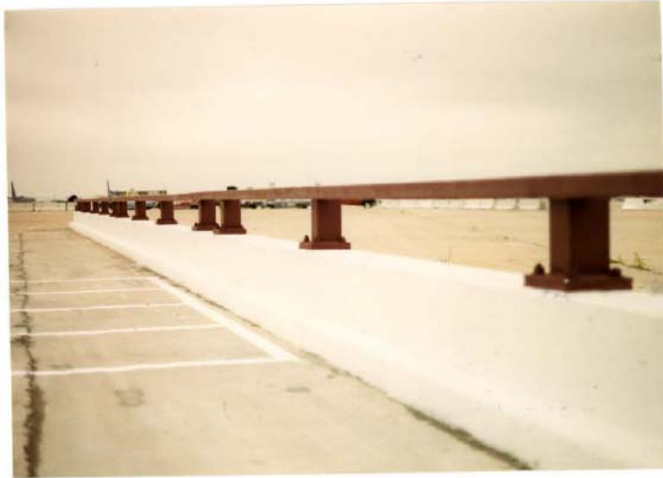
Figure 2. MwRSF test installation of the Minnesota Type Three Combination Bridge Railing. 2
