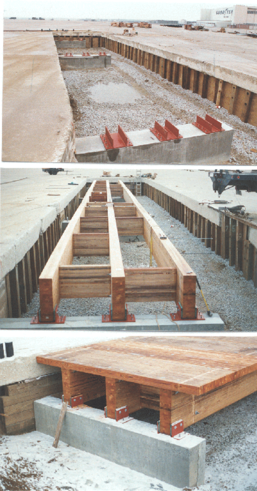
Figure 3. Simulated Test Bridge.
