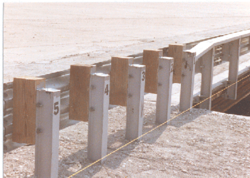
Figure 1. Steel Thrie Beam with Channel Bridge Railing and Thrie Beam with Channel Transition, System No. 1.
