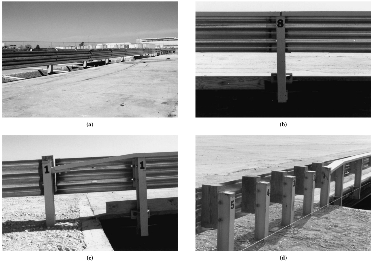
FIGURE 1 Steel thrie beam with channel bridge railing and thrie beam with channel transition, System 1.
