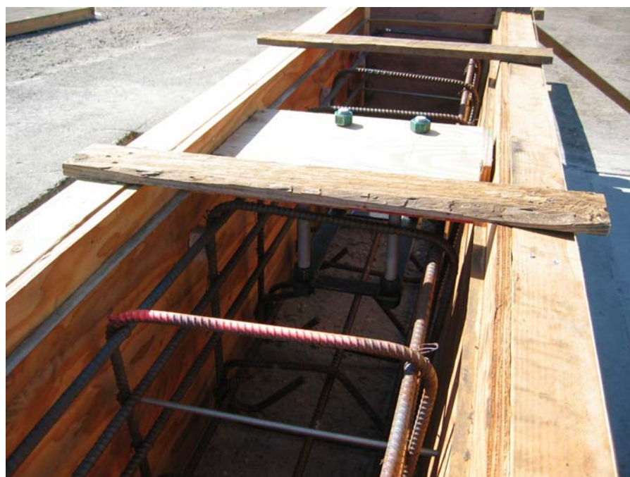
Figure 2-3 – Type 90 formwork in place for the concrete curb
