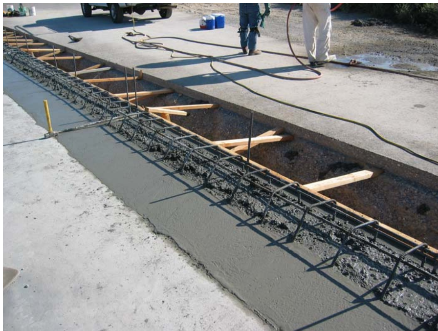
Figure 2-2 – New bridge deck in place for Type 90 bridge rail
