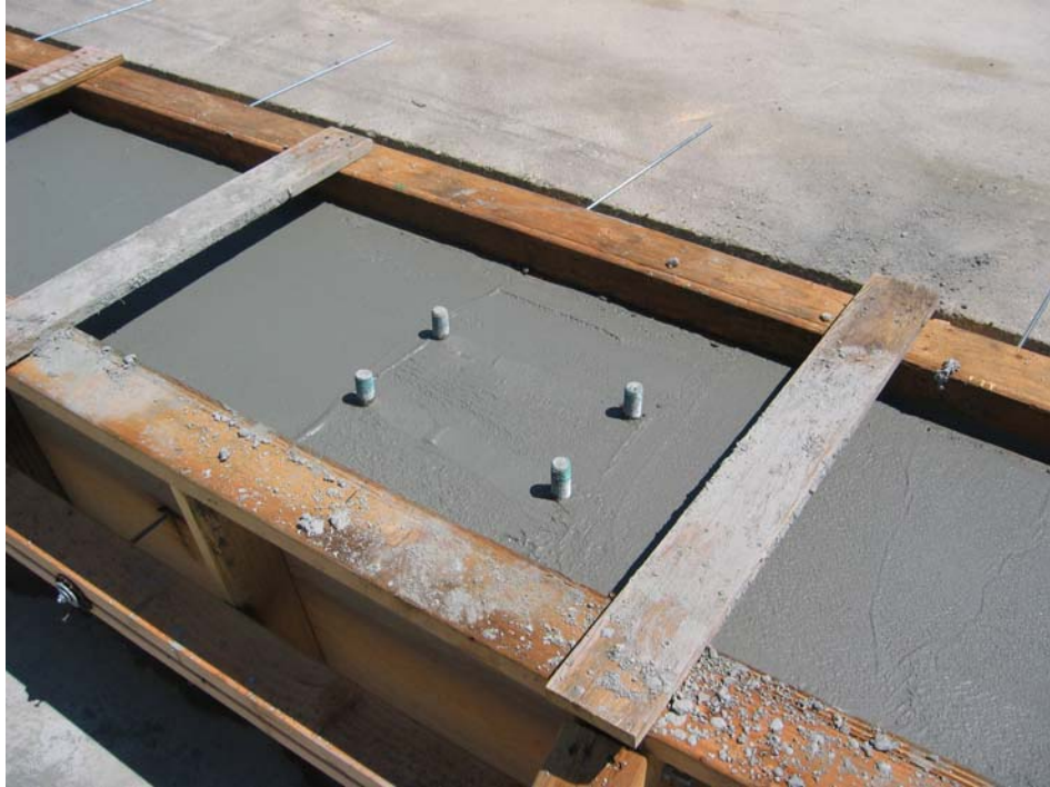
Figure 2-4 – Type 90 concrete curb with cast-in anchor bolts
