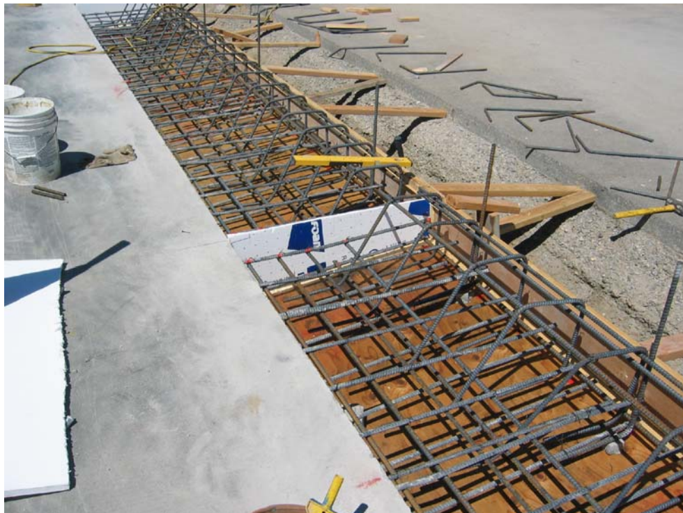
Figure 2-1 – New rebar spliced with existing rebar for new bridge deck
