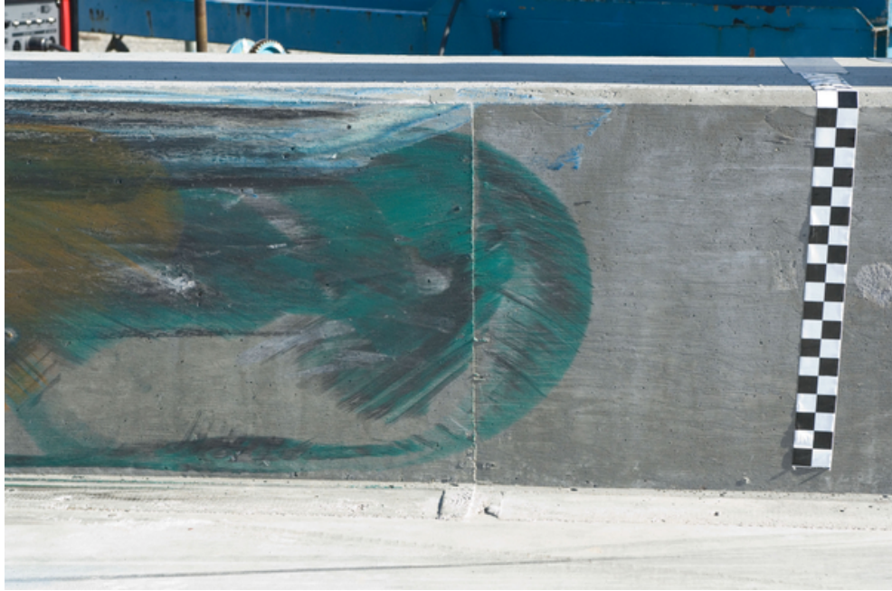
Figure 2-21 – Barrier face scraping after Test 632
