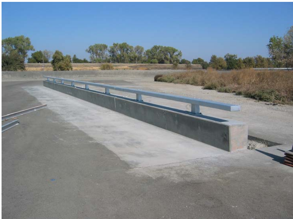
Figure 2-5 – Type 90 with the steel rail in place
