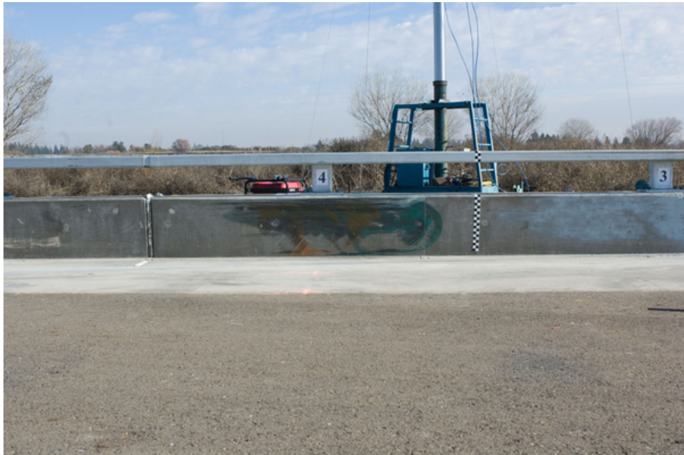
Figure 2-20 – Type 90 bridge rail face after Test 632
