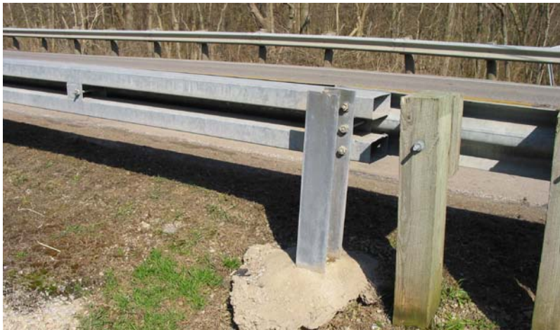
Figure 14: Long-span guardrail across a culvert on HW 315 in Delaware, County.
