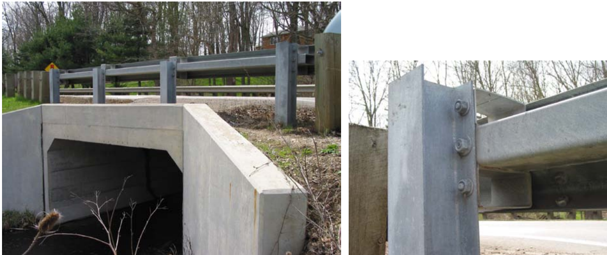
Figure 1: Typical installation of the ODOT GR-2.2 guardrail
