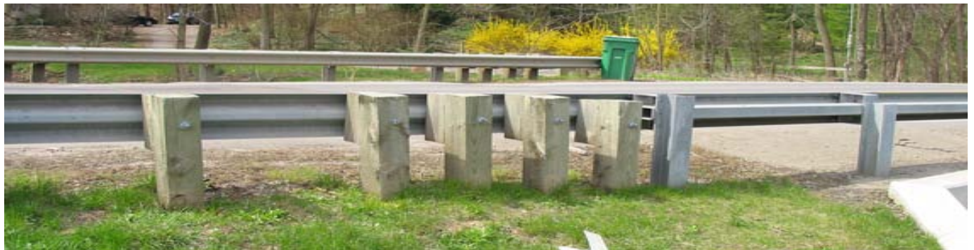
Figure 33: Photo of the ODOT GR-2.2 guardrail and ODOT GR-3.4 transition at a site along HW 315 north of Columbus, Ohio.
